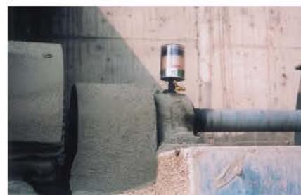
Wind Mill Shaft
